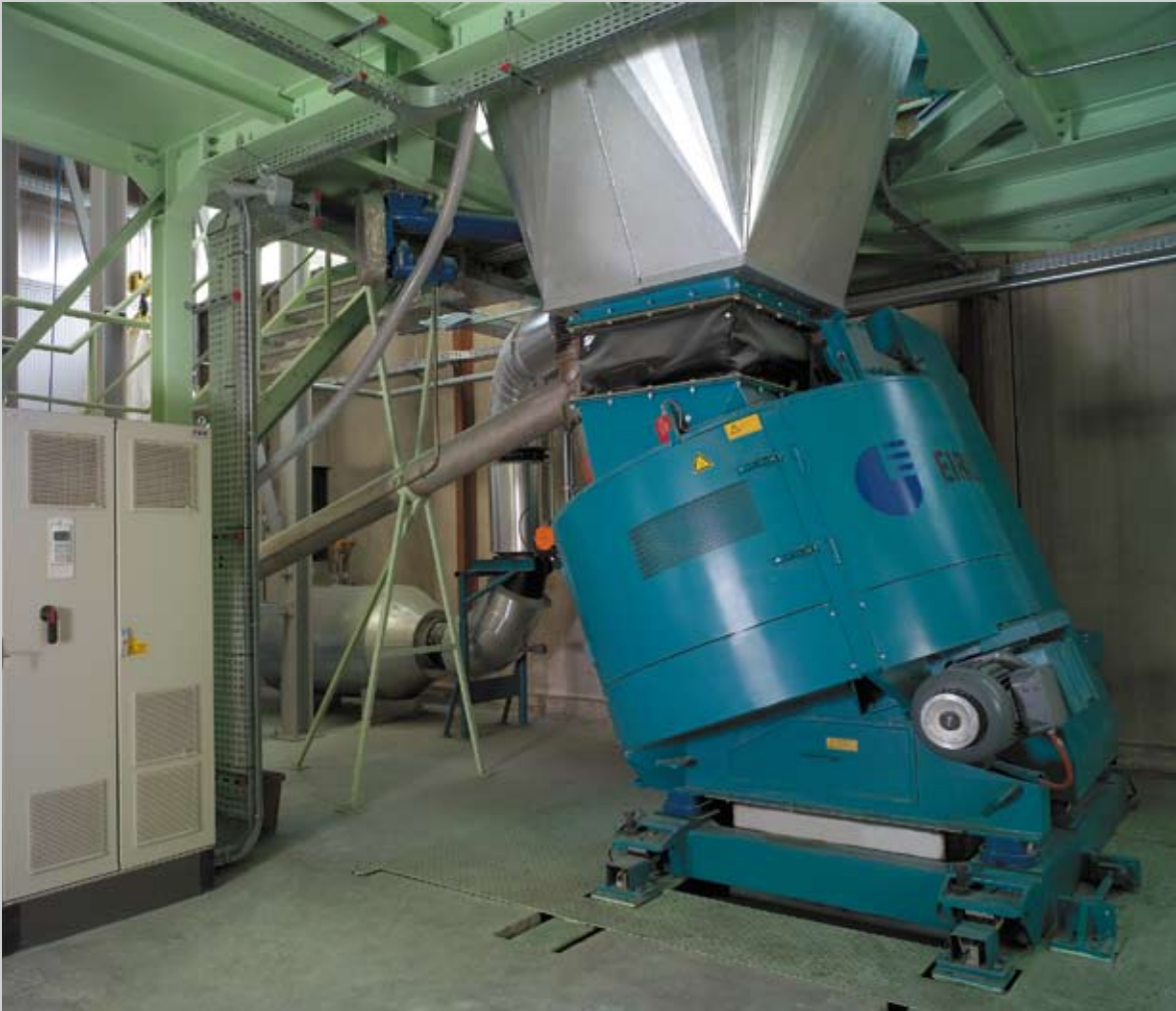
Fig. 7.1: Drying system with gas burner and RV19 intensive mixer
